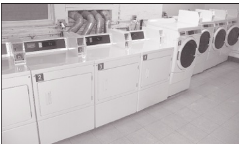
Each building has washers and dryers in the basement.
